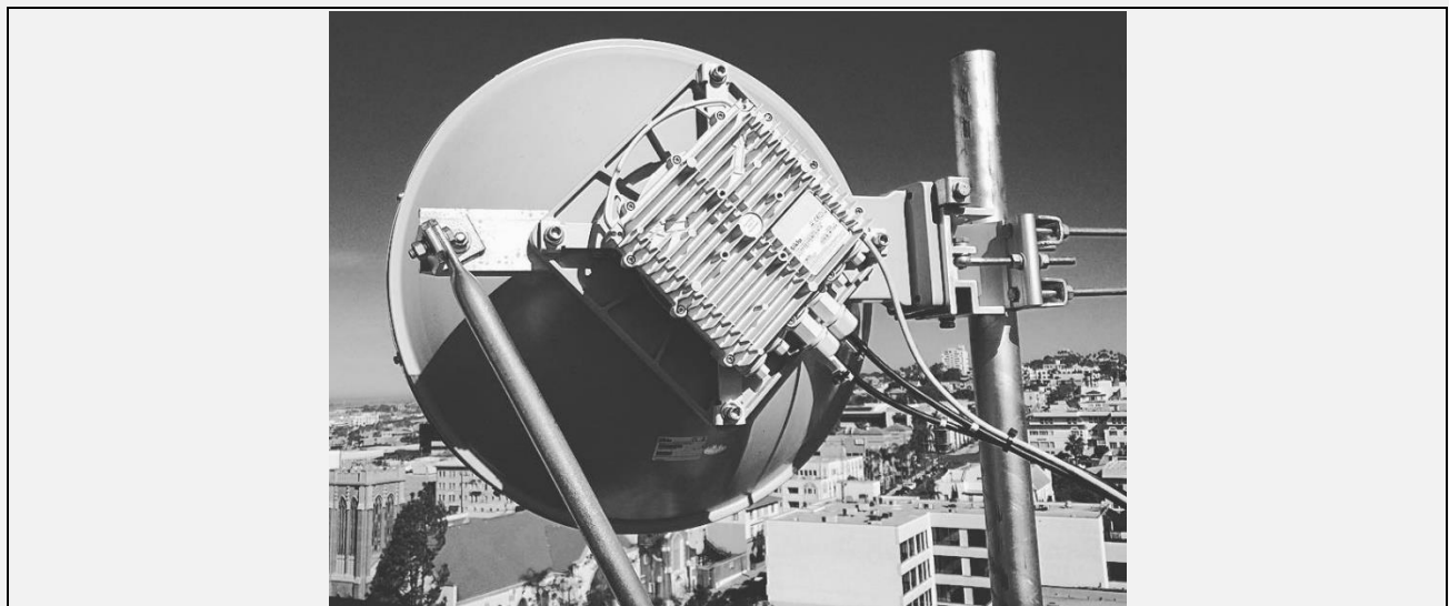
FIGURE 5a: 2FT Antenna installation (EH-ANT-2ft-B)
